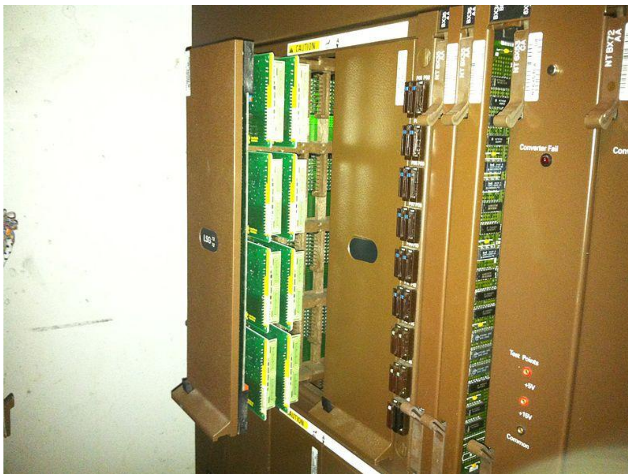
Northern Telecom DMS-100 Line Card Drawer showing line cards
